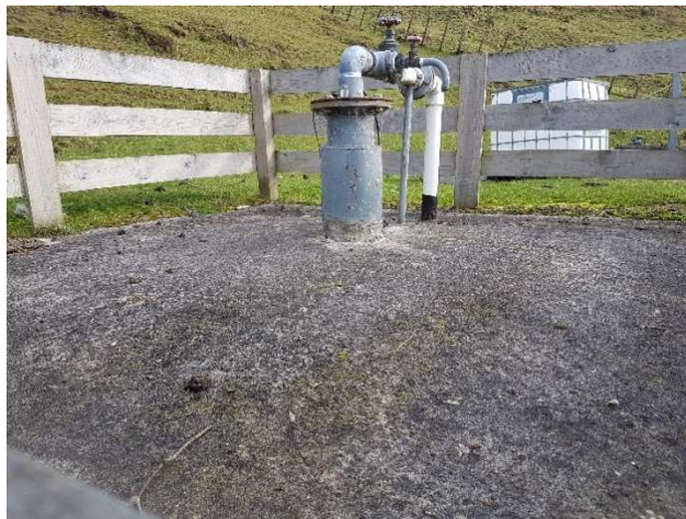
Figure 4. Bore head
