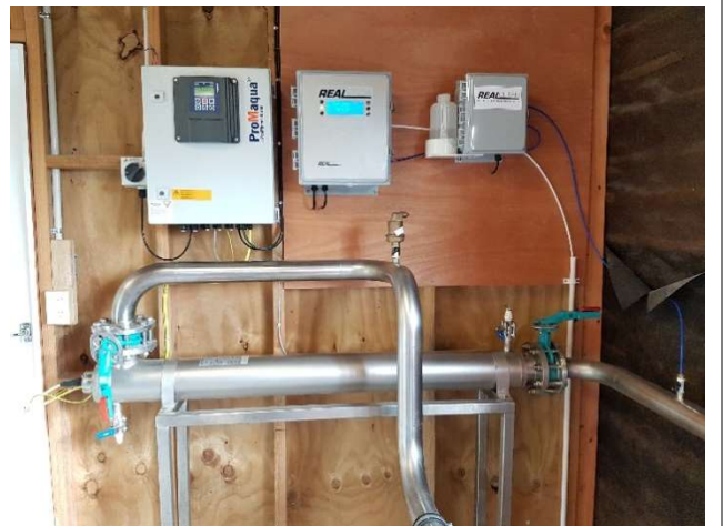
Figure 5. UV reactor
